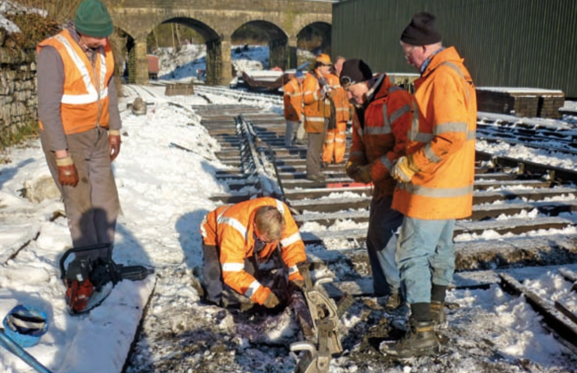
Post Christmas work on the three-way point in the snow - Richard Buckby.
