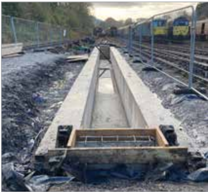
Left: maintenance pit waiting for the steps to be cast.
